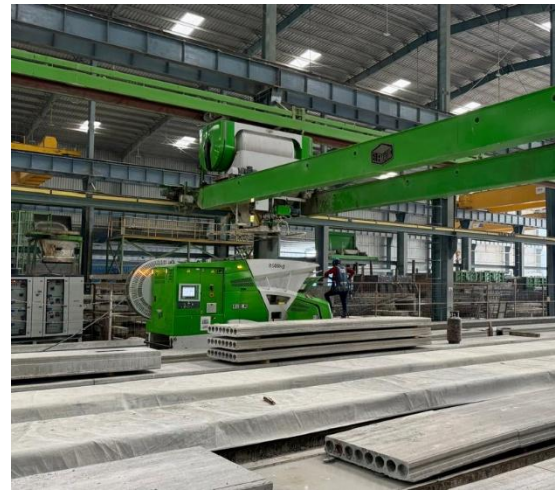
Figure 6b: Concrete pouring for Hollow Core Slabs
