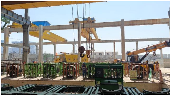
Figure 10: Prestressing strands for casting of slabs
