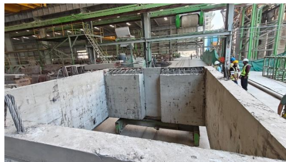
Figure 7b: Precast utility ducts
