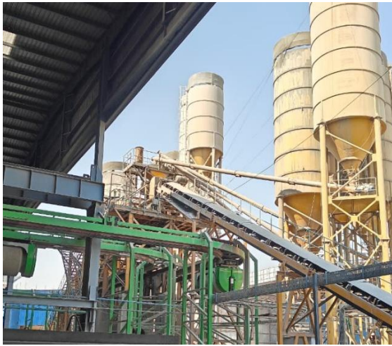
Figure 6a: Concrete Production
